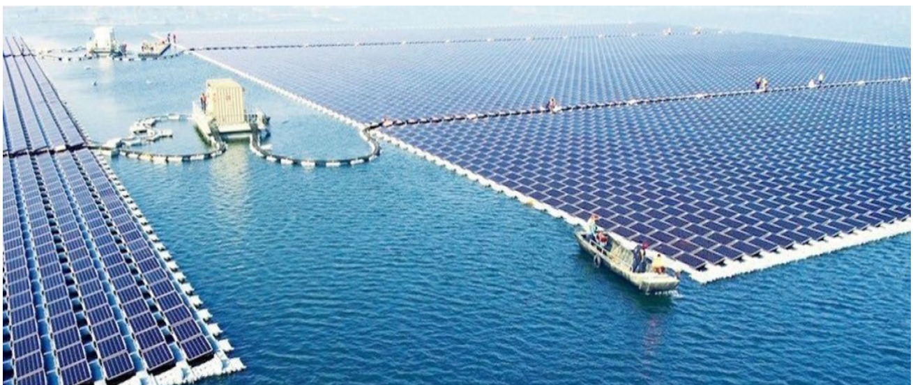
Fig. 1 The world's largest 40 MW floating solar power plant at Huainan, China. (Source: Brandon 2017)
